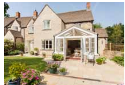
The builders laid the new paving and put up the low wall and fencing to keep safe any future pets
